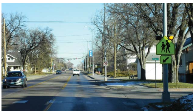
Figure 2.15 – US 26, Two-Lane Highway with Center Two-Way Left Lane Through Morrill, NE
