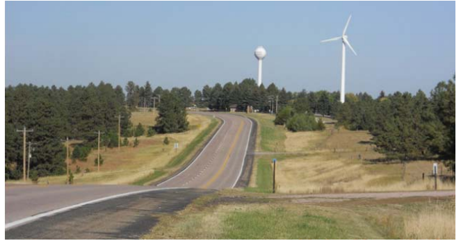
Figure 2.20 – US 385, Three-Lane Highway Through the Nebraska National Forest, Approximately Ten Miles South of Chadron at Mile Marker 157.
