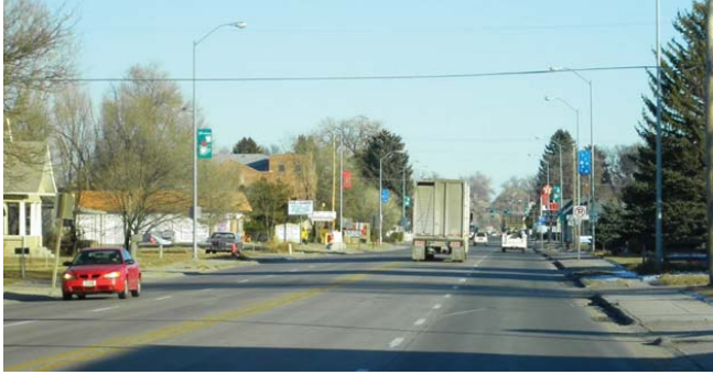
Figure 2.17 – US 26, Four-Lane Highway Through Mitchell, NE
