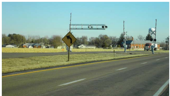
Figure 2.16 – US 26, Four-Lane Divided Highway Entering Mitchell, NE
