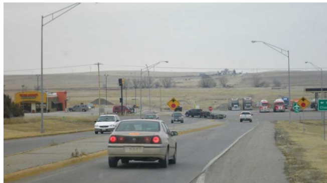
Figure 2.23 – US 385, Intersection at E Jct US 20 and US 385 at Chadron (facing north)
