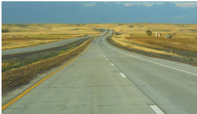
Figure 2.13 – NE 71, Four-Lane Highway Kimball to Scottsbluff
