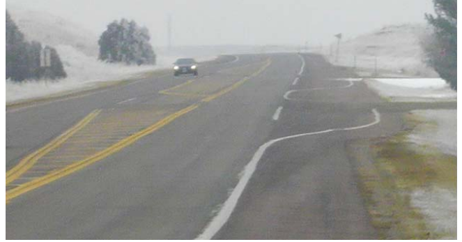
Figure 2.18 – US 385, Two-Lane Highway with Multiple Turning Lanes
