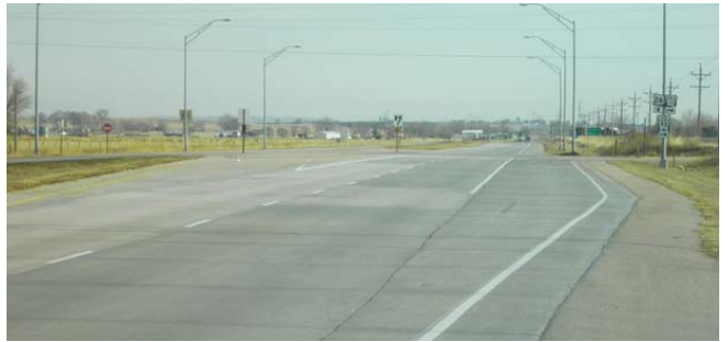
Figure 2.22 – US 26, Intersection of Jct US 26 and NE L79E
